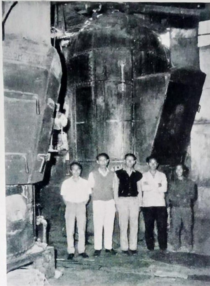
Boiler room with the workers (K.H.P. Hospital, Shillong)
