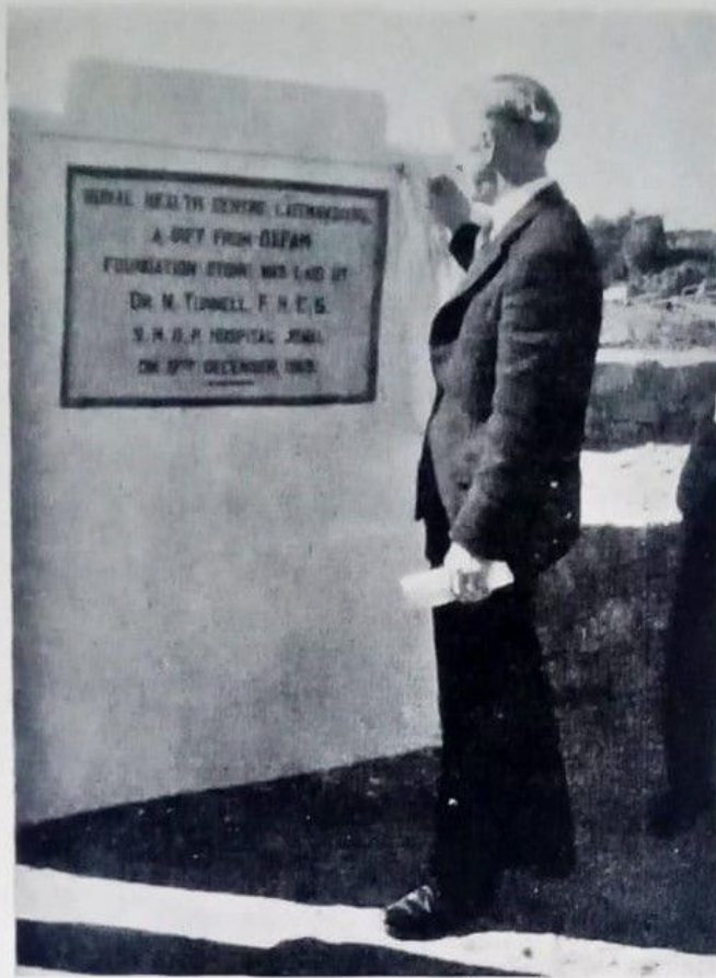
Dr. N. Tunnell, F.R.C.S. laying the foundation stone of Rural Health Centre—Laitmawsiang —a gift from Oxfam
