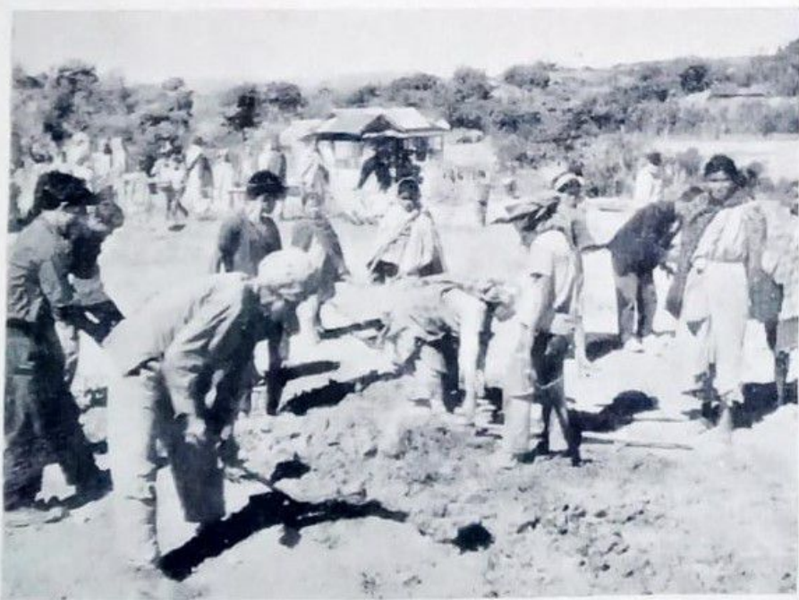
Villagers helping the ground work at Laitmawsiang
